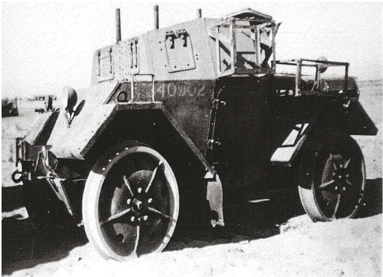
Images courtesy of M Van Alderton Description: Specially converted dingo's, used for patrolling rail lines to check for bombs before the operation of trains. Here can be seen car F340902. Date: Circa 1950's
