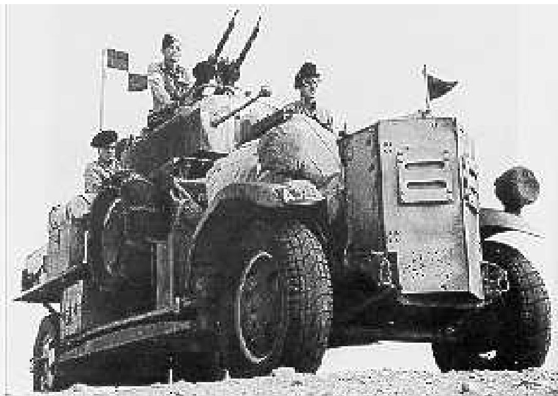
D Squadron, 11th Hussars. Their concern over air attack inspired their use of an extra pair of light machine-guns mounted on the turret.
