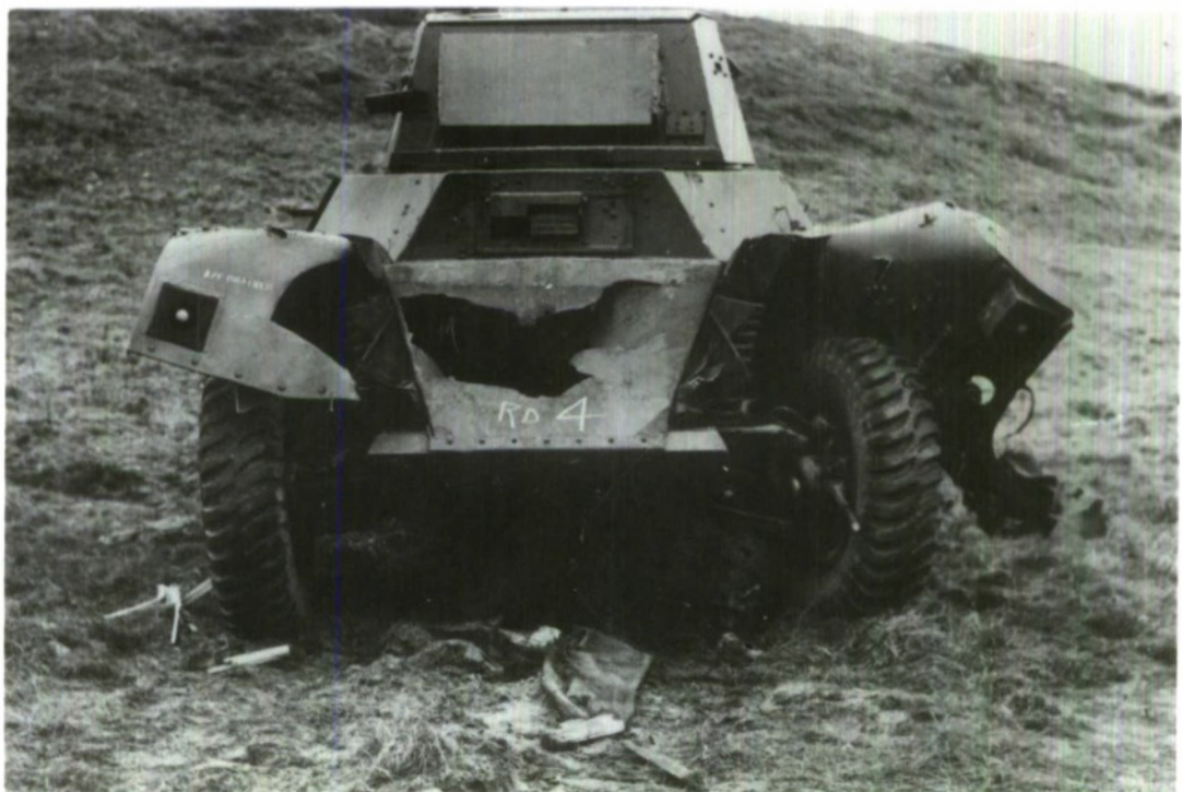
FIG. 9 DIRECT HIT ON CREW COMPARTMENT
