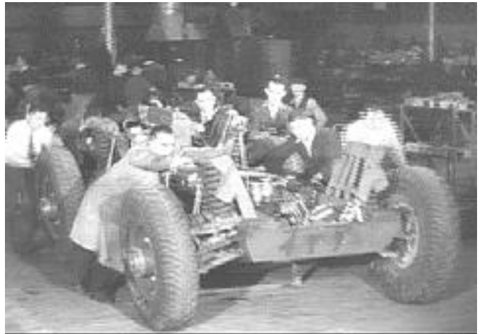
completed chassis and engine assembly
