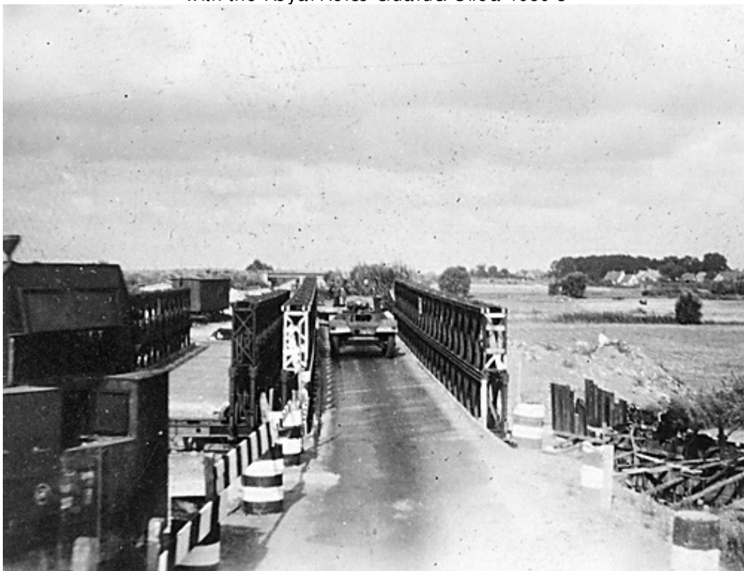
Bailey bridge between Hanover and Brunswick
