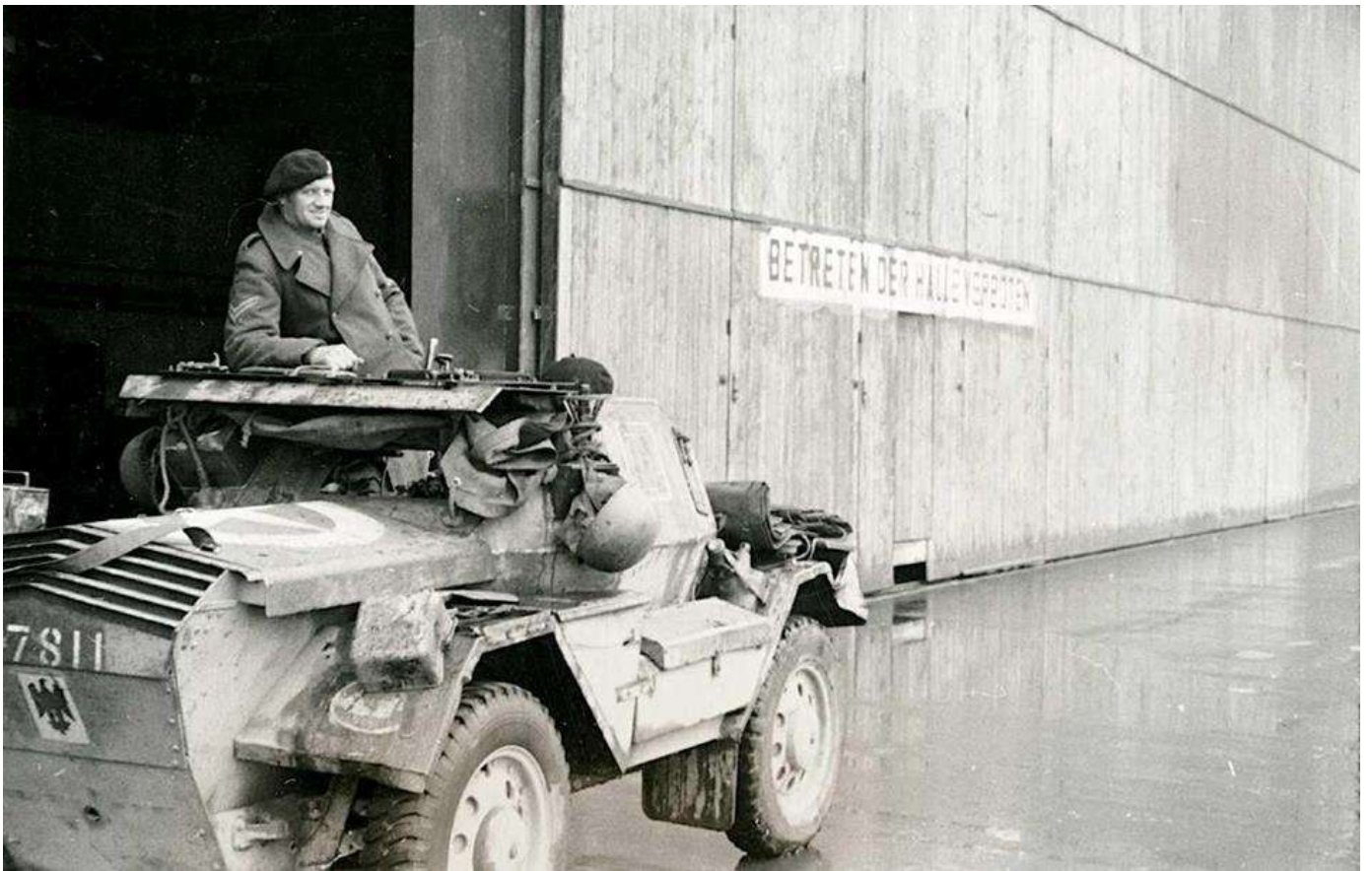
DSC F47811 of the 1st Royal Dragoons aerodrome at Dedelsdorf . the signs says not to enter the building
